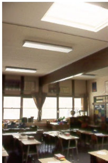
Rogers Elementary with Skylight
