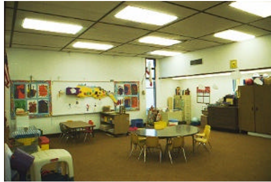
Classroom with Minimum Daylight – Window 1
