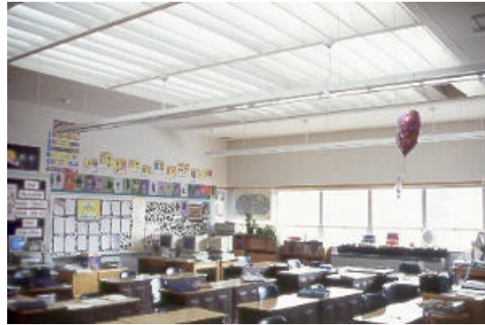
Central Skylight and Diffusing Louvers
