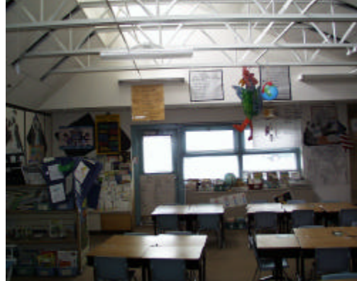
South Facing Monitor Skylights
